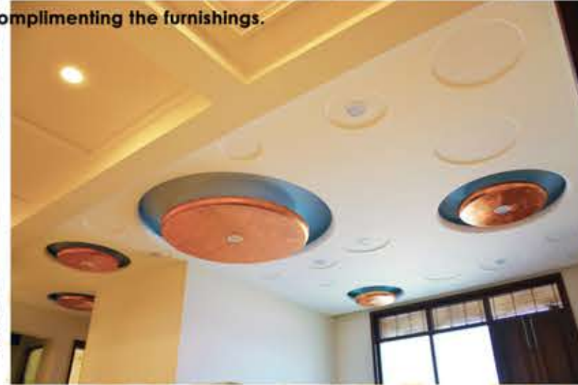
CEILING OF DOUBLE HEIGHT LOBBY IN P.O.P. AND COPPER LEAFING
